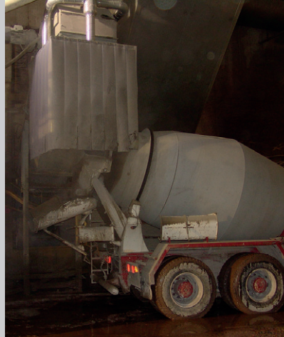
Loading of concrete mixing truck
