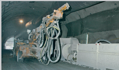
Tunnel Kirchdorf, mobile unit for asbestos
