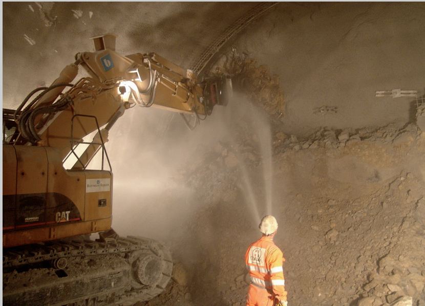
Cutter head, cutting process
