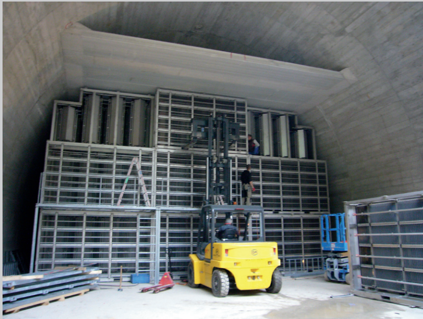
Installation of ECCO filter
